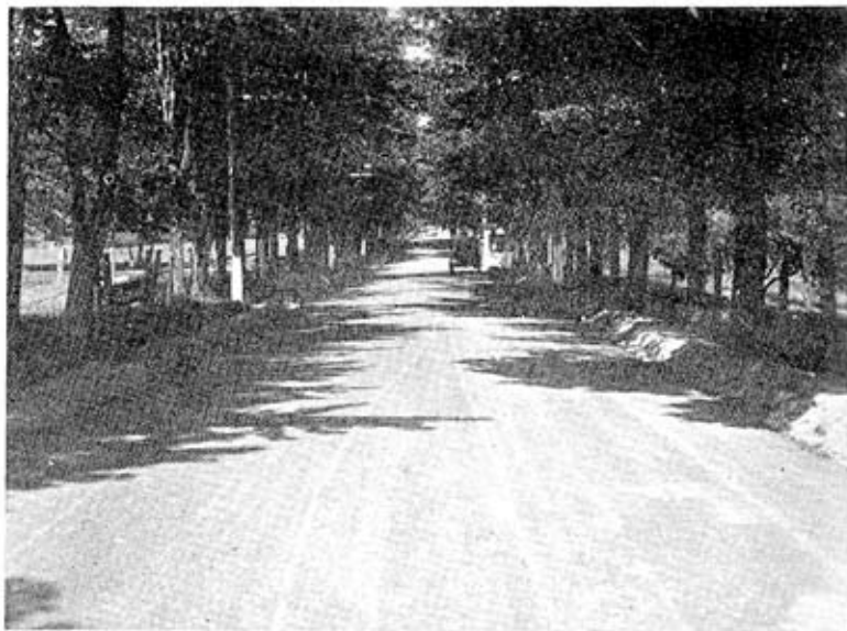
A highway scene at Dewittville, Que. Malone-Montreal Highway No. 4
